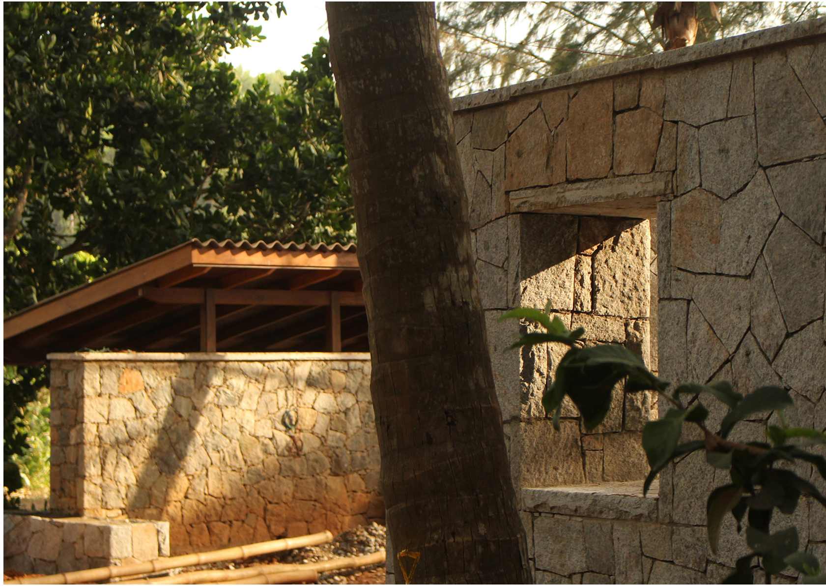
Stone walls surrounding the guest apartment building
