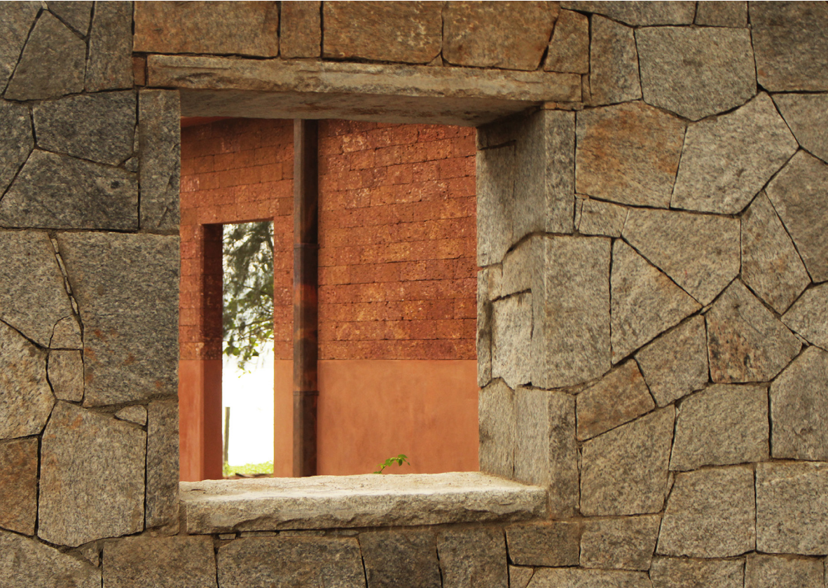
Stone walls surrounding the guest apartment building
