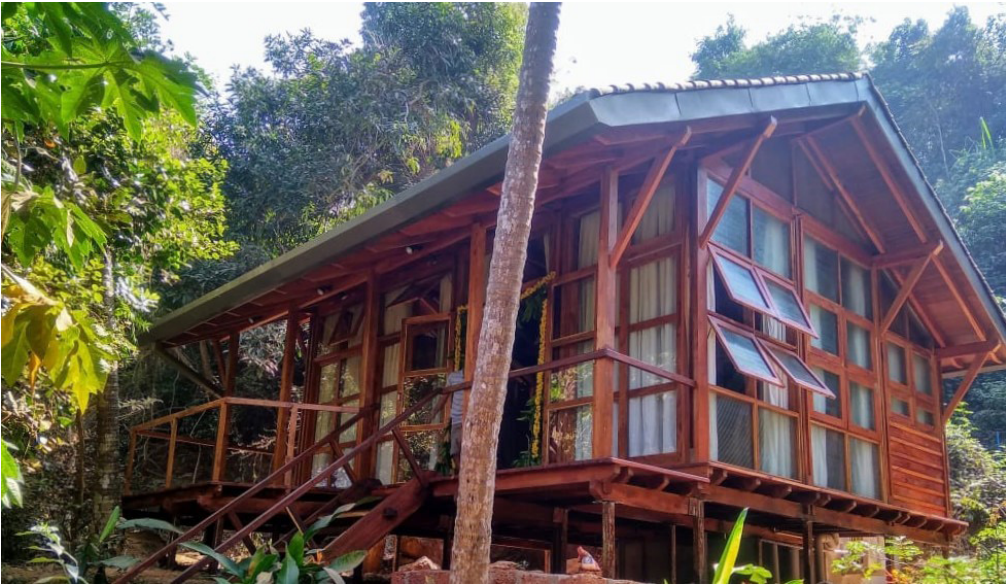
top : Local boatmaker wood working with his indegenous tools and techniques bottom : Wooden cabin protoype raised on Mild steel legs
