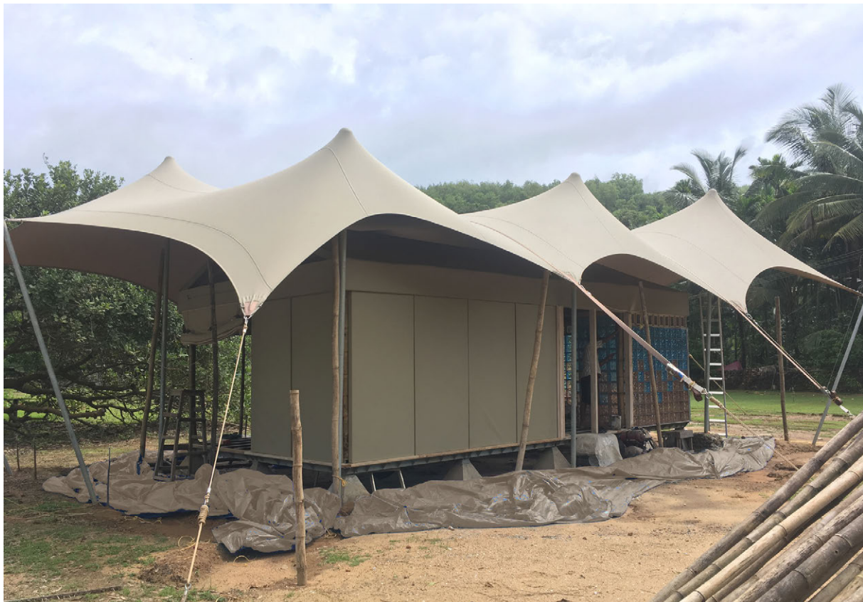
top : dry Assembly of wall panels covered with Rip-stock fabric in progress
