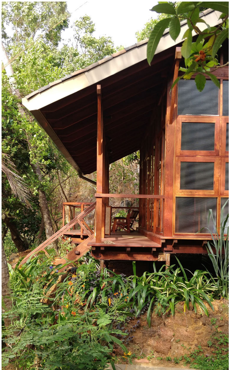
Rainwater harvesting system for watering landscape
