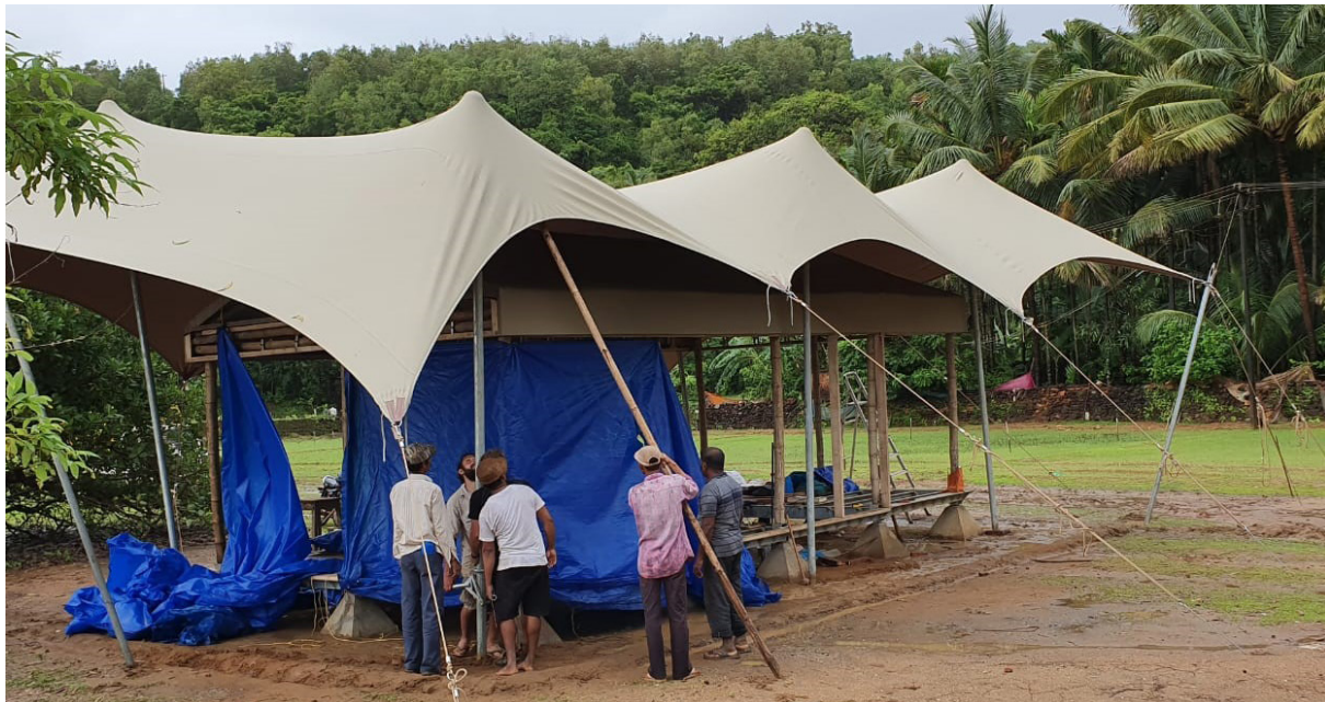
top left & bottom : Local craftsmen raising the tensile structure in collaboration with engineers from South Africa
